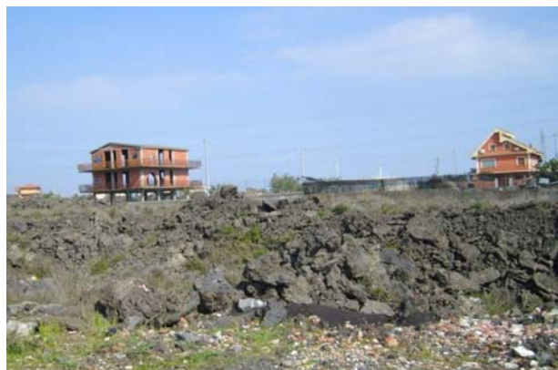
Fig. 2 – Illegal buildings on lava soil in the north part of Catania
