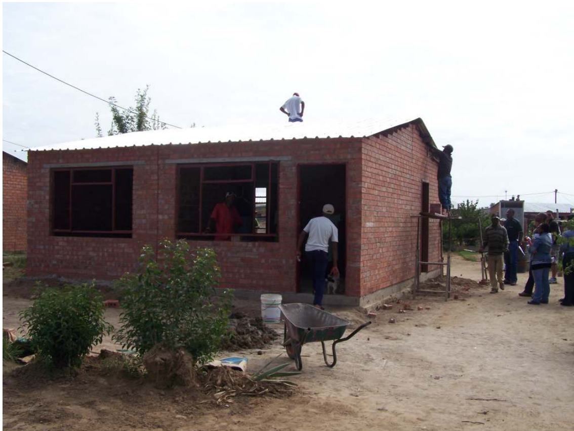
A photo of a nearly completed PHP house. Source authors (2008).
