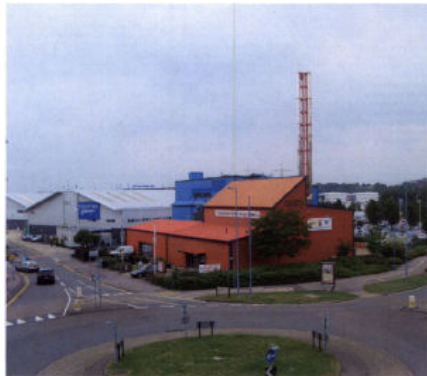
Photograph by J. Jenkison. Southampton geothermal and CHP Station.
