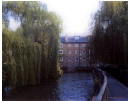
Photograph by J. Jenkison. Wharf Mill direct flow hydro proposal. Itchen River, Winchester.
