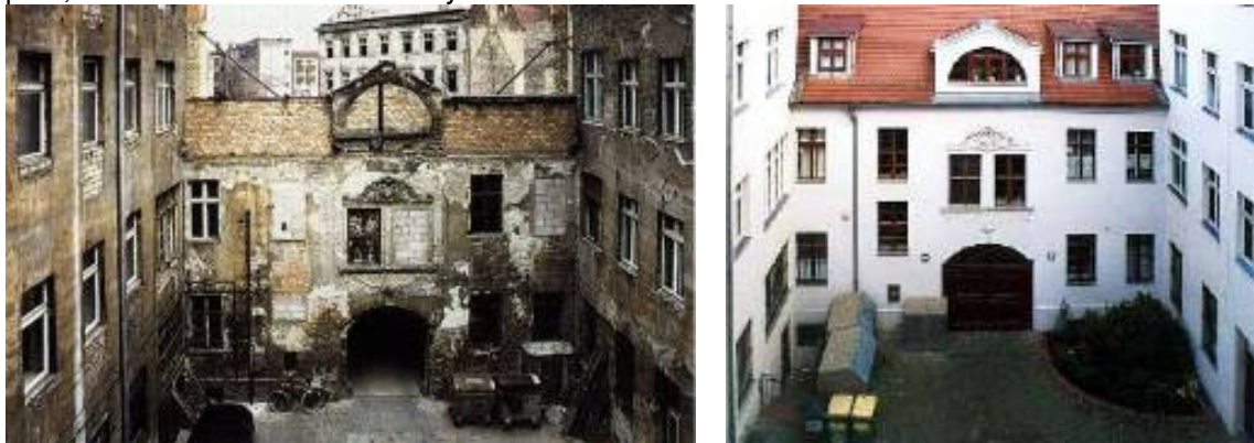
Figure 4: Gips Street 11 before and after restoration
