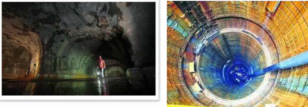
Figure 10: Jurong Rock Caverns (Source: JTC)
