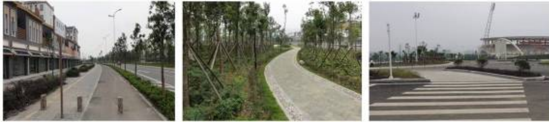
Figure 3: Implementation of non-vehicular transportation and traffic calming concepts: vehicle blocking stone, pedestrian-bicycle lane, and pedestrian island, CAUPD
