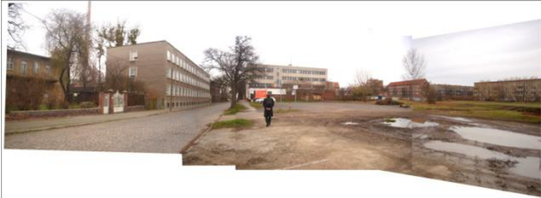
Fig. 1.1: Apartment buildings, vacant dwellings and wasteland in Dessau, photos source: Silja Tillner
