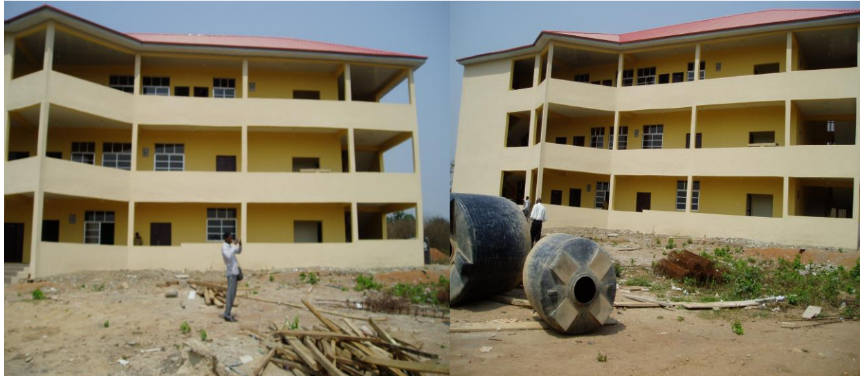
Figure 5: New ISOP Building Planned and Designed by Students
